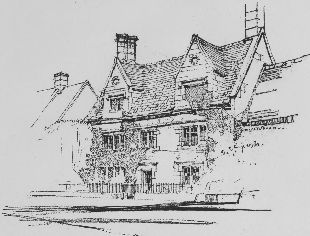
BROADWAY (WORCESTERSHIRE) LIMESTONE WALLS ROBSTONE ROOF.
